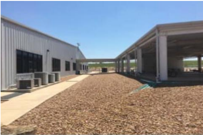
Main Building & Pavilion Exterior
